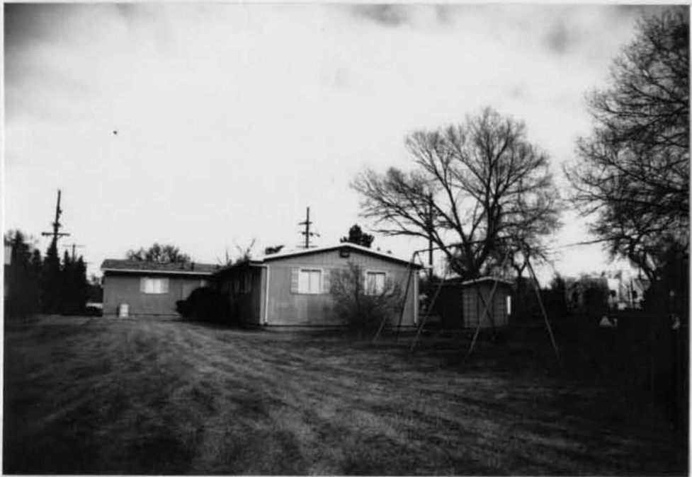
1997 Modular Bldg. View to North
