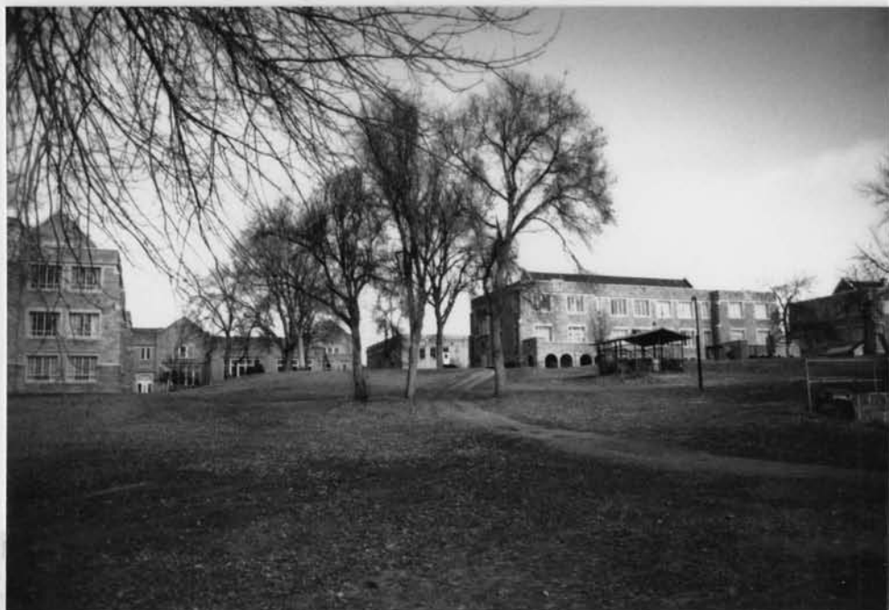
1997 Brown, Ritter, Argo View to Northeast
