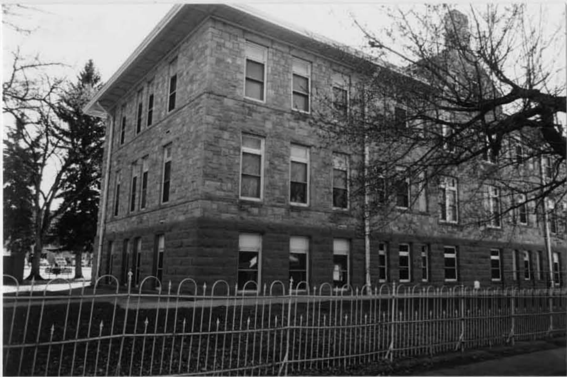
1997 Jones Hall Northeast face
