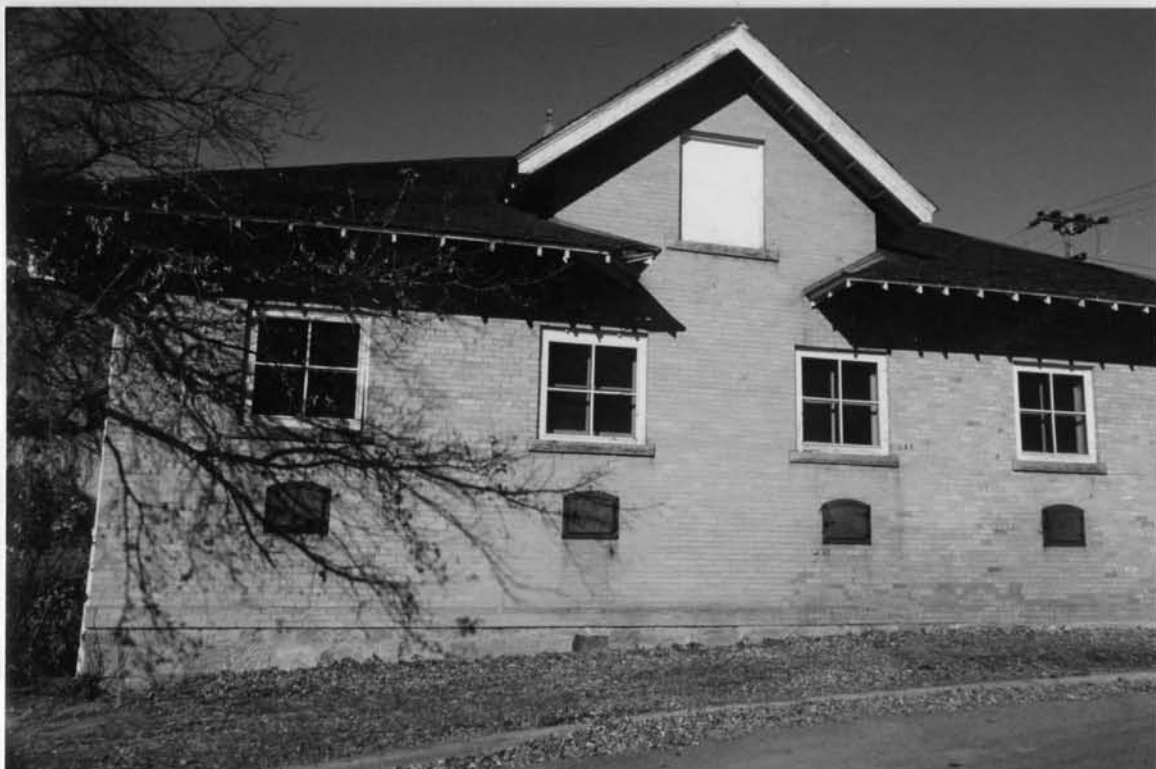
1997 Barn south face
